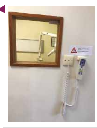
Figure 21. Example of lead glass window enabling the observation of the patient during imaging. The lead glass absorbs the stray X-ray radiation.
